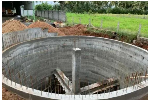
Figure 2 Circular Water Tank
