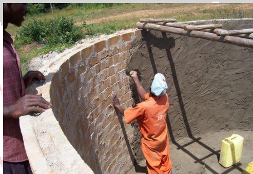
Figure 1 RCC Circular Underground Water Tanks
