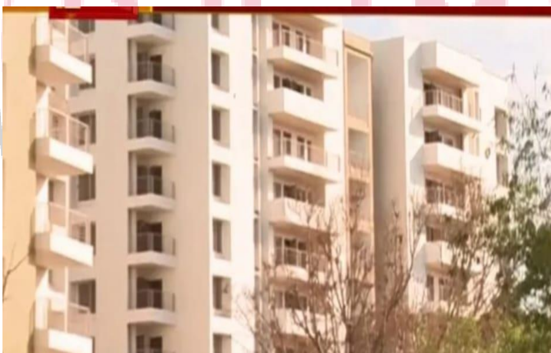
Figure 3 Site Picture of Block A
